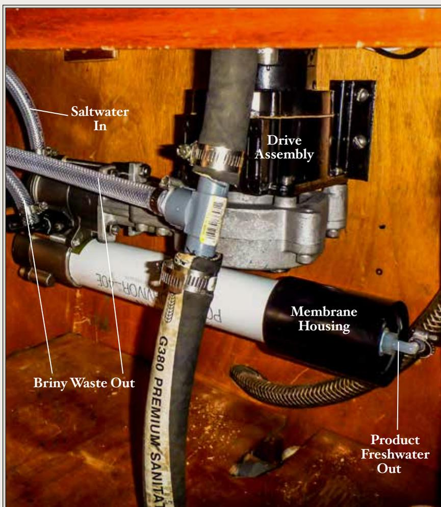
The drive assembly and membrane housing are the heart of every watermaker system, and some of the largest components. The membrane housing must be positioned horizontally. In the installation above, the briny discharge hose comes out of the membrane housing and makes a loop to tie into the boat's sink drain.
