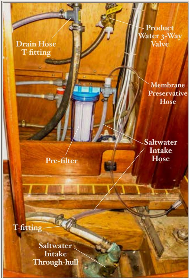
**T-fittings were used to tap into the boat's starboard tank fill plumbing, saltwater intake hose and sink drain (left), so Ellen and Seth didn't need to add any through-hulls. A three-way valve mounted ahead of the pre-filter (right) adjusts to allow the input of either seawater or membrane preservative to the system.**
